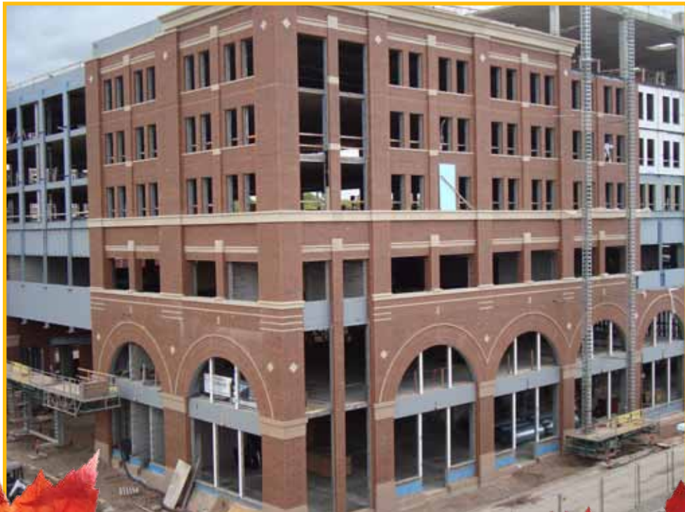
Grand River Station – transit center in Downtown La Crosse under construction
