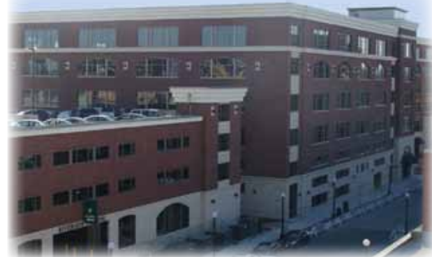
The $19 million Riverside Center III and the $12.5 million Riverside Center parking ramp opened this fall. The Riverside Center ramp features 535 parking spaces and the office facility hosts an additional 328 parking spaces.
