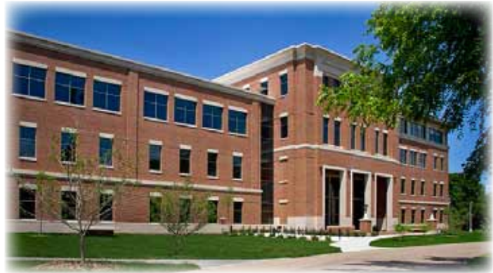
UW-La Crosse's Centennial Hall academic building was dedicated this fall just as students were returning to campus. This $44 million project provides 44 new classrooms and lecture halls. Eagle Hall residence hall also opened to students this fall. Photo courtesy of Sue Lee, UW-La Crosse.
