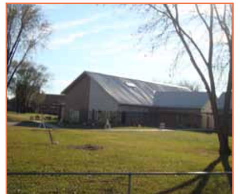
The new Black River Beach House Community Center will serve as a wonderful community asset on La Crosse's Northside.
