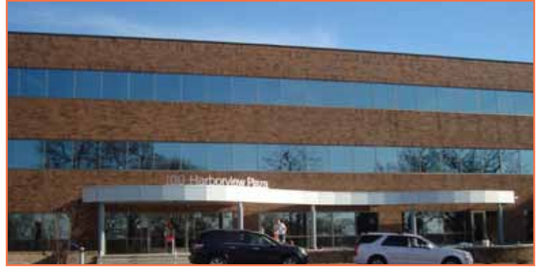
Remodeling of the 48,000 square feet 100 Harborview office facility is nearing completion.
