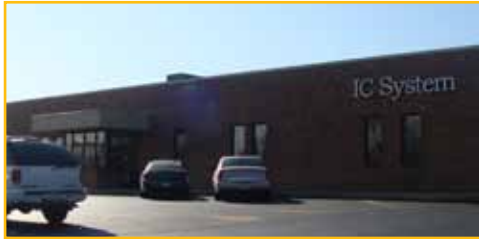
I.C. System's new facility at Center 90 in Onalaska
