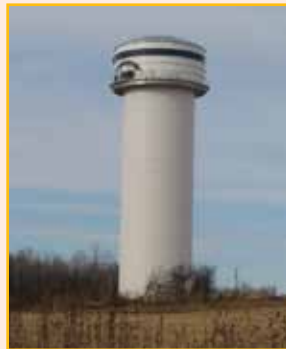
New water tower in Lakeview Business Park will provide service to park tenants and the Village of West Salem
